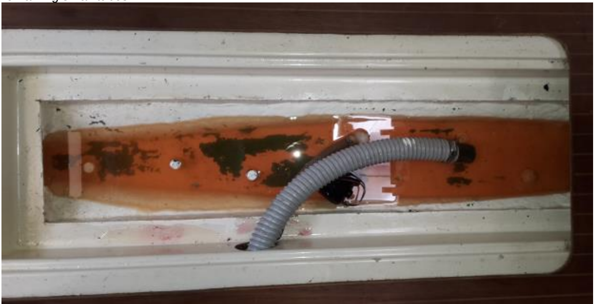
Image 2 Bilge with oily water - nobody wants to see this.
